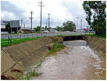
Stormwater in a conventional engineered drainage channel. Source: Bidgee (CC)
